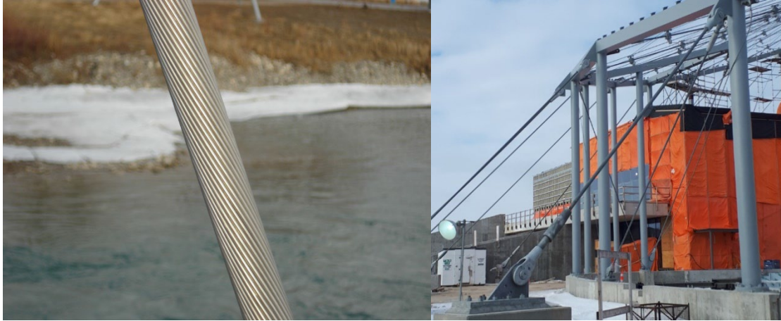
Figure 1. Stay cable as installed in a bridge in Calgary, Canada and in a building under construction in Winnipeg, Canada (Authors Photos)
