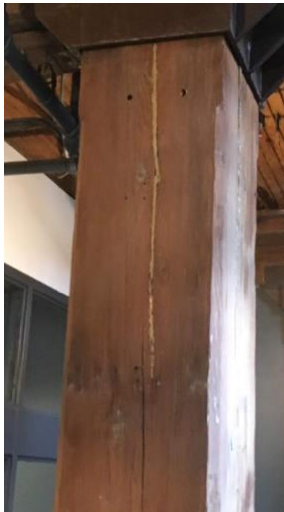
Figure 1. Partial attempted sealant repair on a radial crack present on a column.
