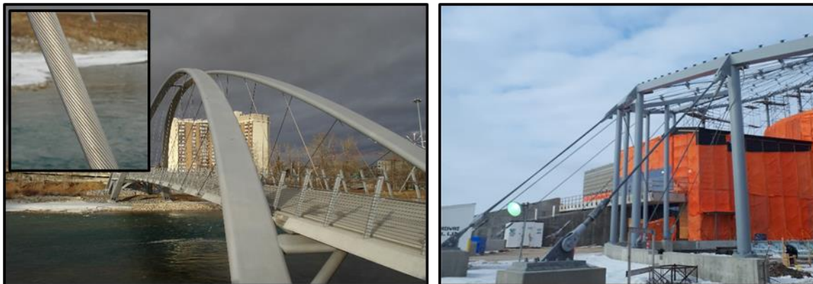
Figure 1.2. (Left) A cable-supported bridge in Alberta, Canada with an inset photo of a steel cable member; (right) a cable-supported structure in Manitoba, Canada.
