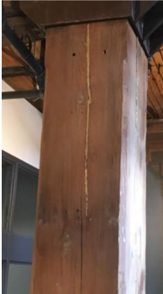
Figure 4.1. Partial attempted sealant repair on a radial crack present on a column.
