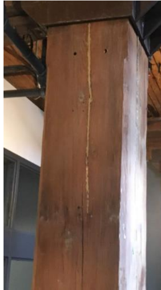
Figure C.1 Partial attempted sealant repair on a radial crack present on a column (author's photo).
