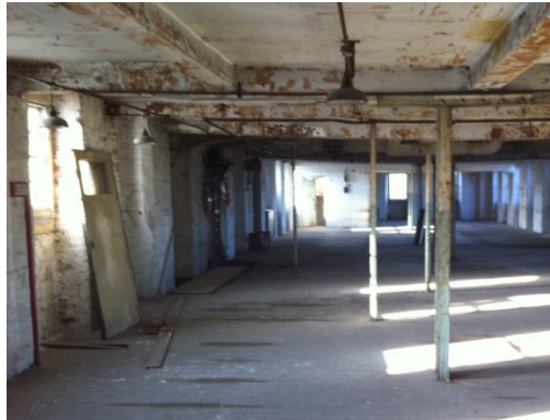
Fig. 1. Metallic plates installed since the 18 th century structure, believed to make the structure incombustible
