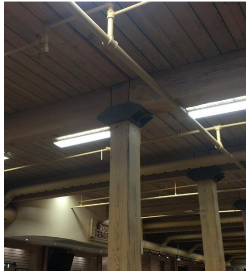
Fig. 3. An exposed timber building, with a timber ceiling, as well as timber beams and columns connected by a cast iron cap. This structure is located in Toronto, Canada, and was constructed in 1902 as a warehouse (but is currently being used for commercial retail purposes)
