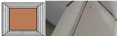
Figure 1. Encapsulation installation procedure of a stand-alone column (prior to gap sealing/wall-finishing), representative of encapsulation used in Canadian tall timber structures
