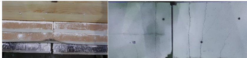
Figure 17. Post-fire 'seam' opening in Column 3
