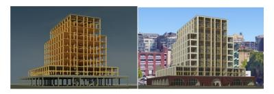
Figure 1: Structure of *Hypothetical A* engineered timber hybrid building (left), and exterior of *Hypothetical A* building (right).
