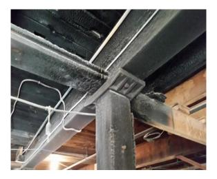
Figure 4. An arson attack on heritage timber where the smaller timber beam components had significant damage, whereas the larger column had minimal damage as the core cross-section remained (authors' photo).
