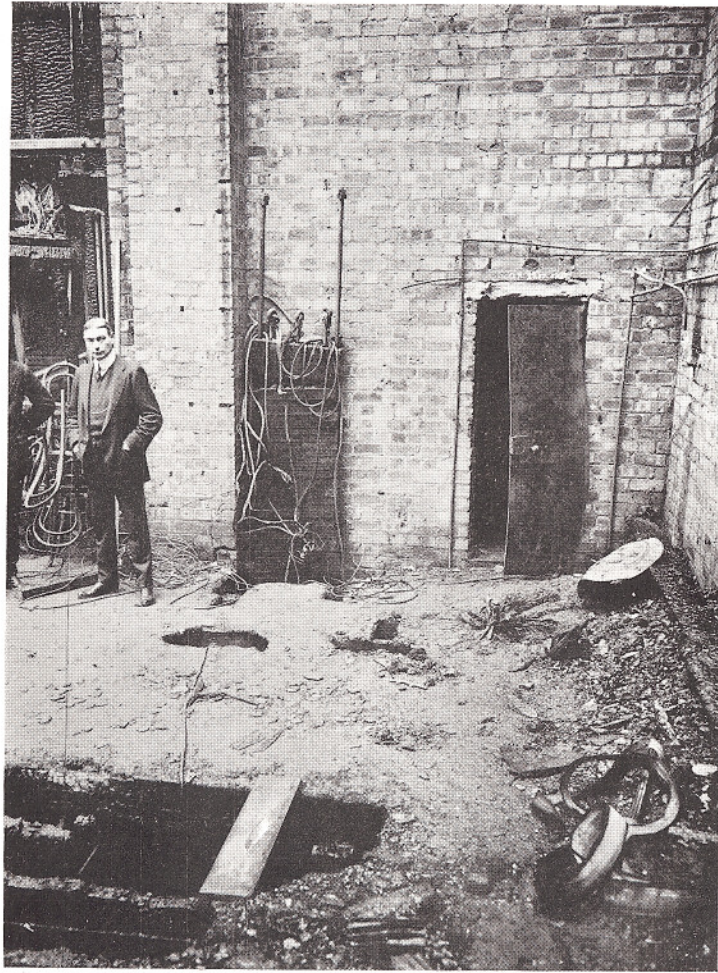
Fig. 15 View of the O.P. side of the stage showing the iron pass door to auditorium and the curtain counterweight.
